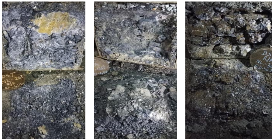
Fig. 3. Jointed blocky dolomite at Kuri Gongri HE Project
